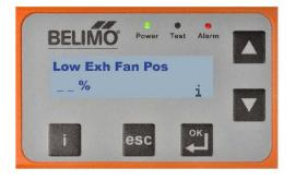
LOW EXH FAN POS = SET % OF ECONOMIZER O/A DAMPER OPEN THAT WILL ENERGIZE POWER EXHAUST WHEN BLOWER FAN IS RUNNING AT LOW SPEED
